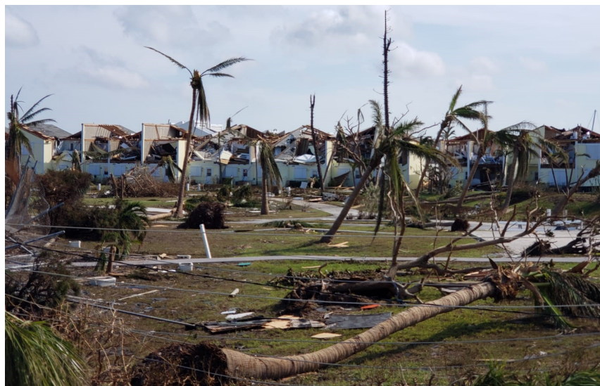
For this publication, we again utilised photographs such as this one provided by Father DeAngelo Bowe, Rector of the Holy Spirit Anglican Church in The Bahamas, which show the immense damage caused by Hurricane Dorian in 2019.
